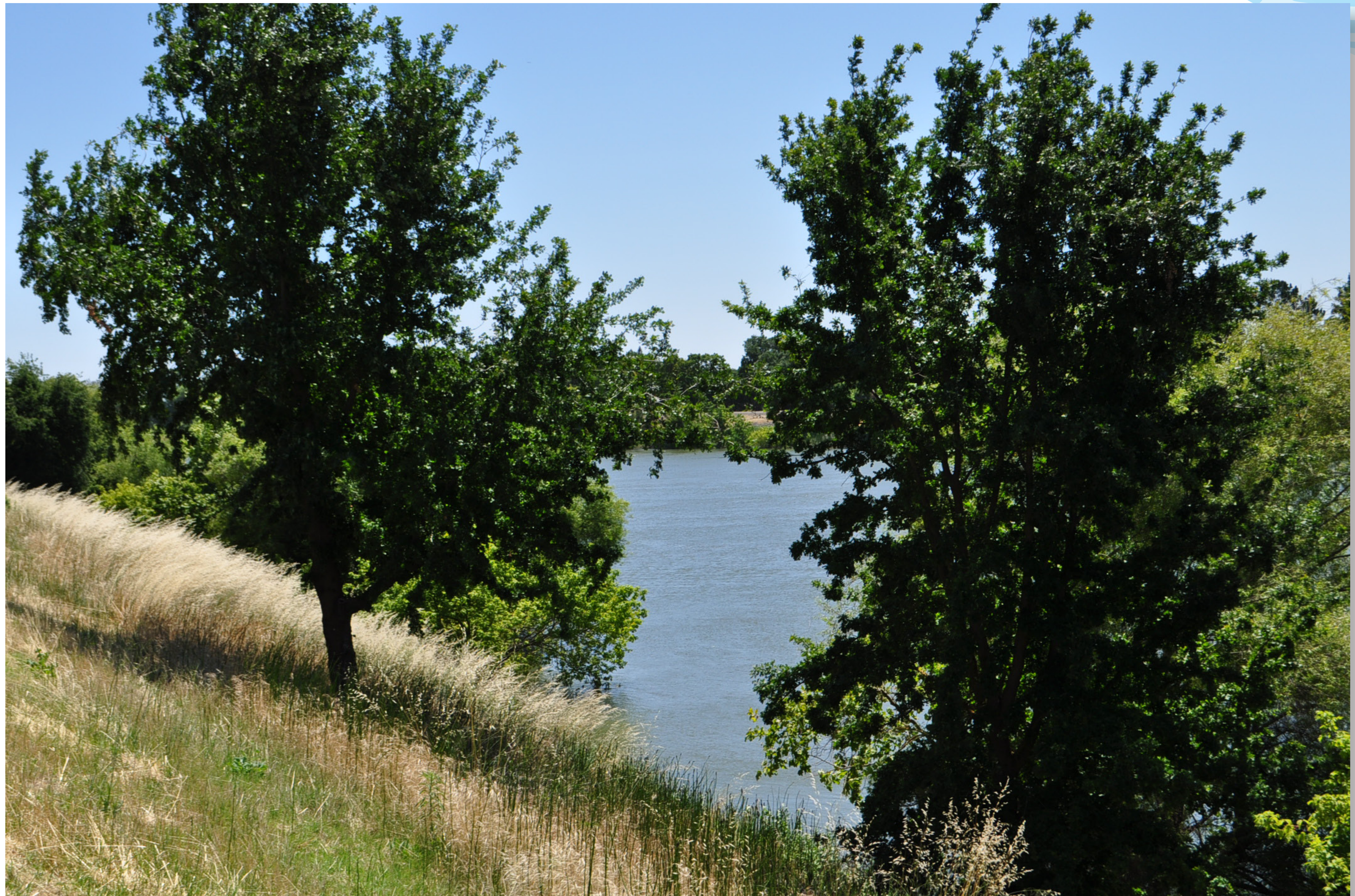
On South River Road, looking east and across the river toward Sacramento's Little Pocket neighborhood. This levee stretch is included in the 6.4 miles proposed for upgrades under the Southport Sacramento River EIP.
