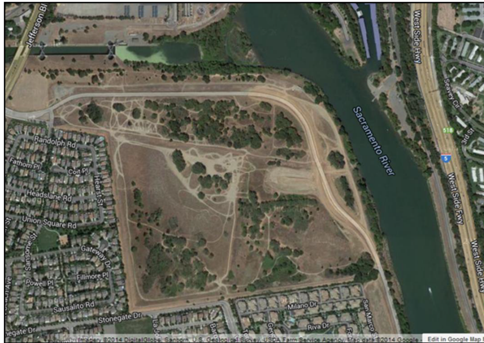
Fig. 4. Construction of the setback levee at the northeast corner of the WSAFCA EIP bordered by the Barge Canal on the north, Sacramento River on the east, and Jefferson Boulevard on the west. Work on the project began on April 6, 2011 and 3 years later, the 2,200 foot long setback levee has not yet been completed. The vacant area in the figure was created on the east by the setback levee, on the north by the barge canal levee, and on the west and south sides by existing levees. Off road vehicles, dirt bikers, paint ballers, hunters, and horseback riders have severely eroded trails into the area that is posted with no trespassing signs. Squatting by homeless people and illegal dumping is common. The closure of the South River Road to construct the setback levee has created a haven for drug dealers and crime due to isolation caused by the absence of regular traffic. An intent of the setback levee project was preservation of wildlife habitat, but few desirable native plants and wildlife find sanctuary in the vicinity.
